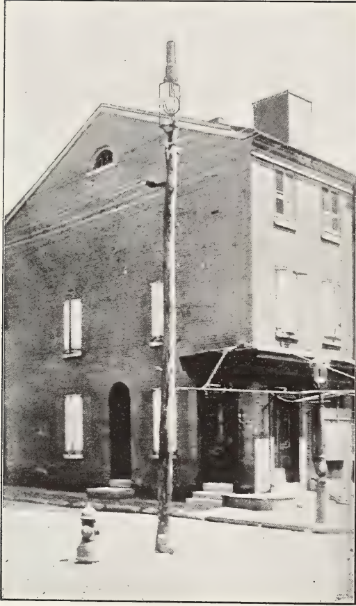
Shows building as it originally stood.
